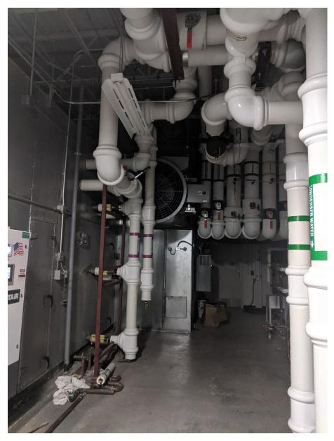
{Differential pressure controls allow unique flow to different areas. This fan is controlling distribution flow. Treated air is pushed to each area at specific rates.}
