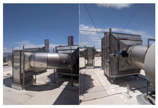
{Air exhaust is diverted though two HEPA filtration units before discharge to the atmosphere.}
